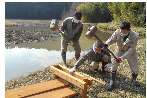
Building a wooden path
