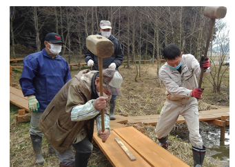
Building a wooden path
